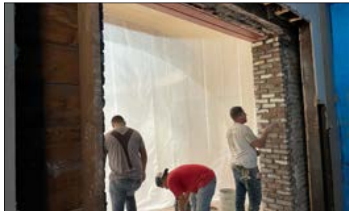
Workers opening passage between McGivney & Reising Ballroom.
